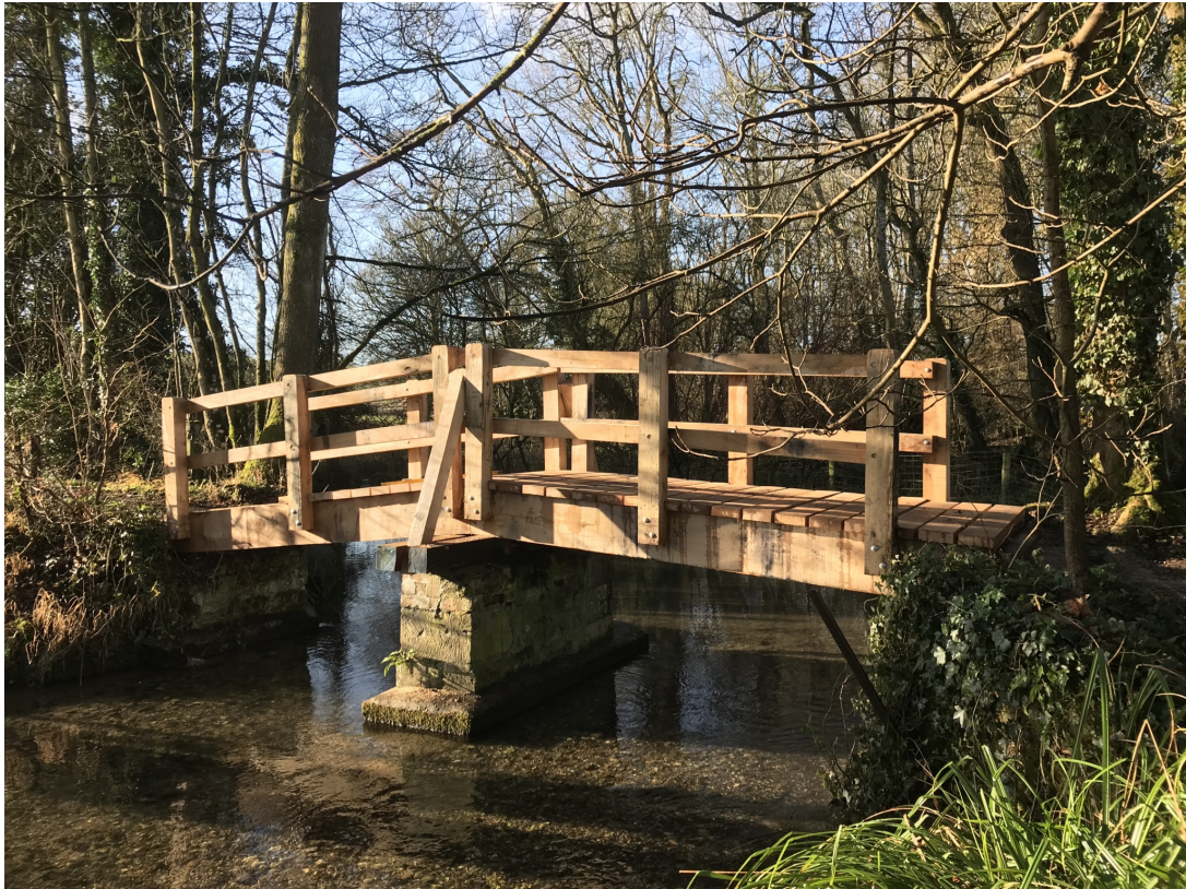
Figure 6: The new footbridge at the ford in Kingston Deverill
